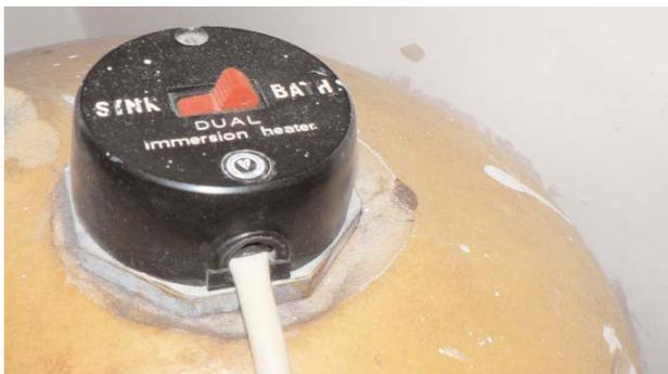
Older immersion heater without thermal cut-out
