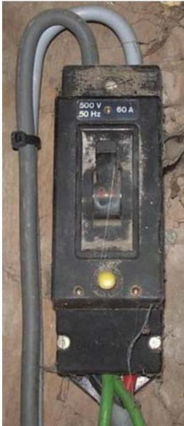
60 A voltage-operated earth-leakage circuit-breaker.
