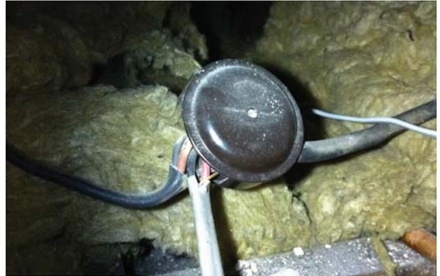
Cable sheaths not taken inside non-conducting enclosure
