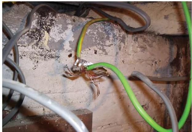
Absence of a reliable means of earthing
