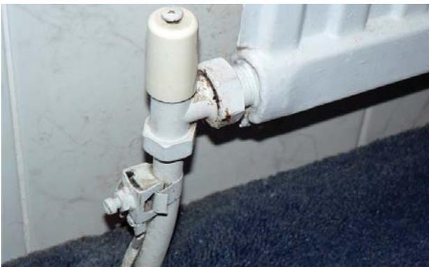
Unmarked bonding conductor
