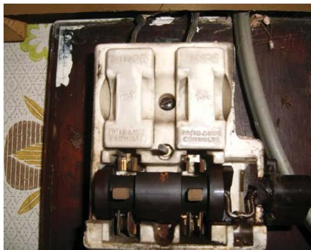
*Double-pole switch with fuses in each pole*
